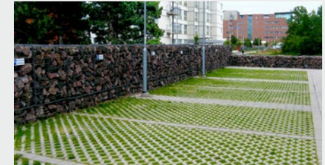
Permeable Parking Surface, Stockholm, Sweden
